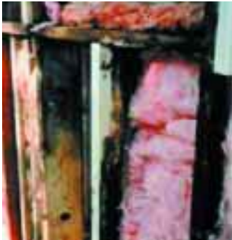
It takes only a small amount of consistent moisture to create problems in a wall.
