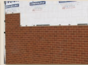
Panel Installation - Newport Brick™ - Red-Buff
