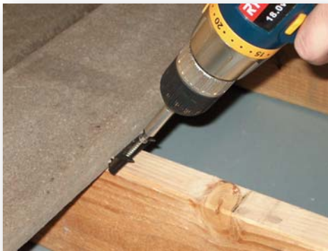
Install decking screw through Tiger Claw fastener, securing it to the support.
