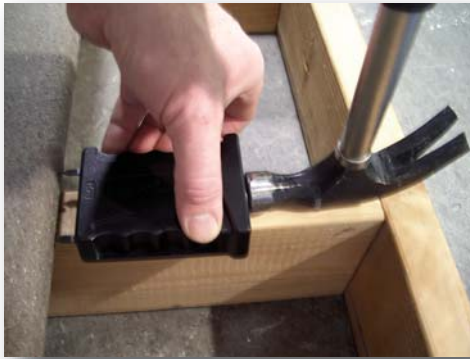
Simply drive Tiger Claw into decking edge using installation block provided.
