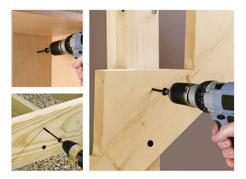
HeadLOK should be installed using a high torque, 1/2" variable speed drill (18V if cordless). Drive the HeadLOK head flush to the surface. No predrilling required when proper end and edge distances are maintained.
