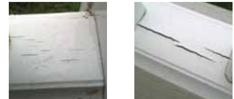
Above shows small cracks that turn into large cracks.
