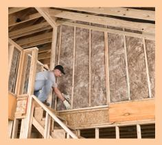
**EcoBatt insulation is naturally brown**— assures no phenol, formaldehyde, acrylics or artificial colors are used in the manufacturing process.
