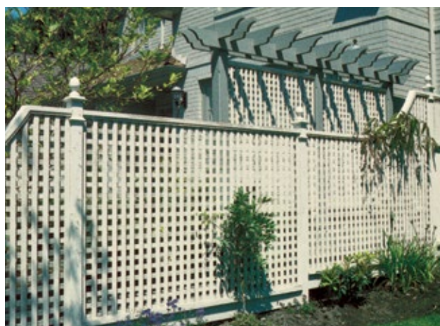
A simple post and rail lattice fence. Finials on posts add a distinctive touch.
