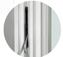
Casement locking mechanism
